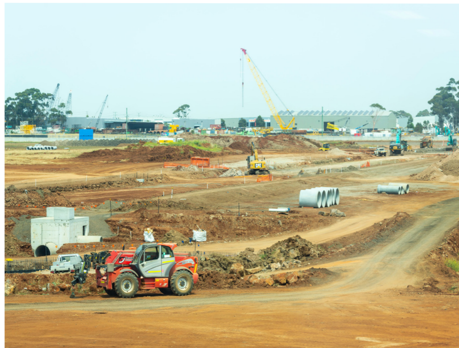
Above: Infrastructure project in Africa
