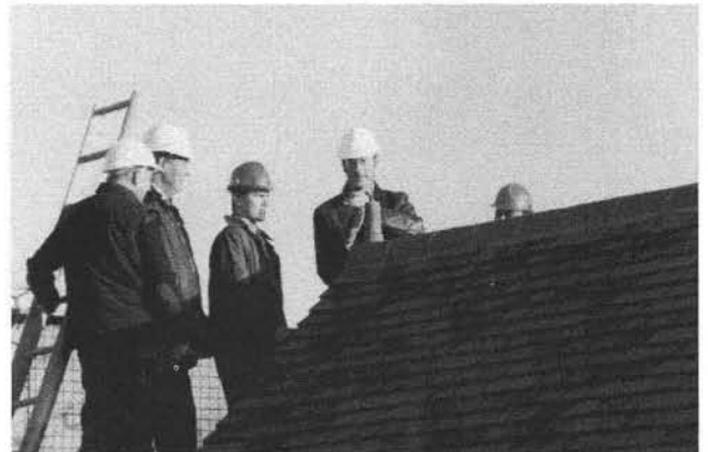
2. The "Top" is inspected...
