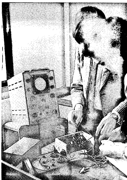
Final checks on the E.C.G. Amplifier
