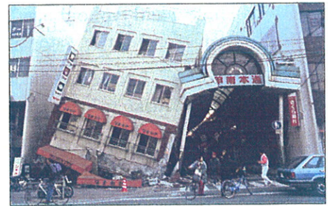
▲ Fig 2 Collapsed building in Kobe.
