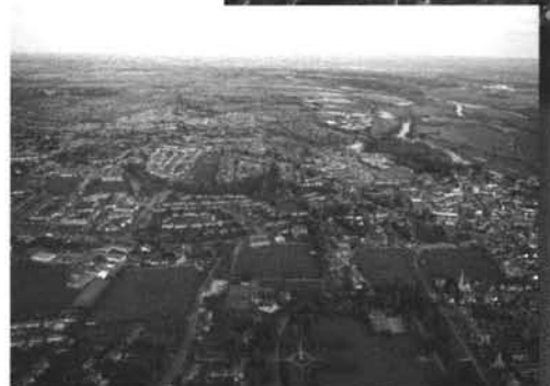
Looking east towards Nuneham Courtenay
